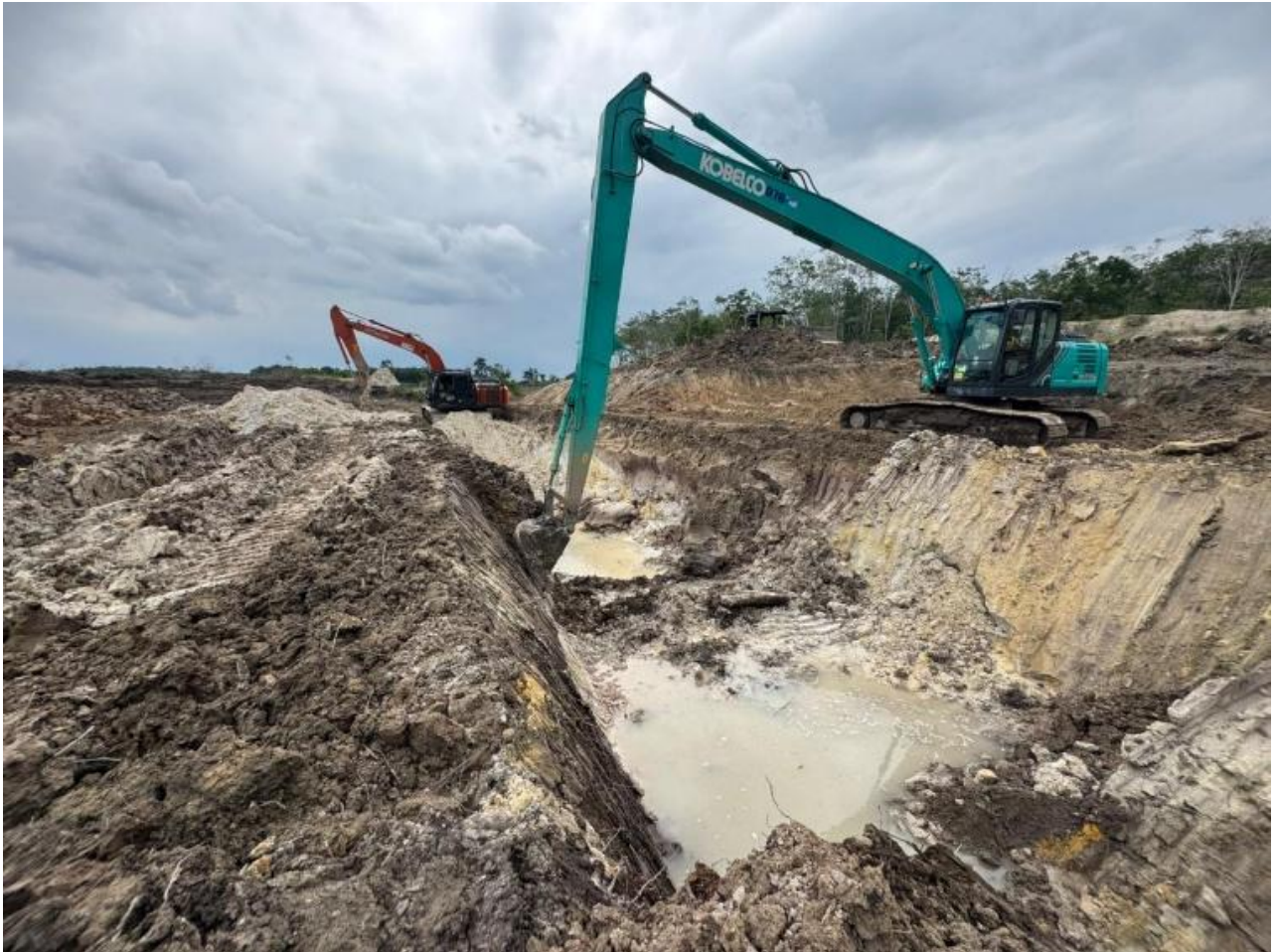
Lampiran 1 Galian Box Culvert STA 69+560
