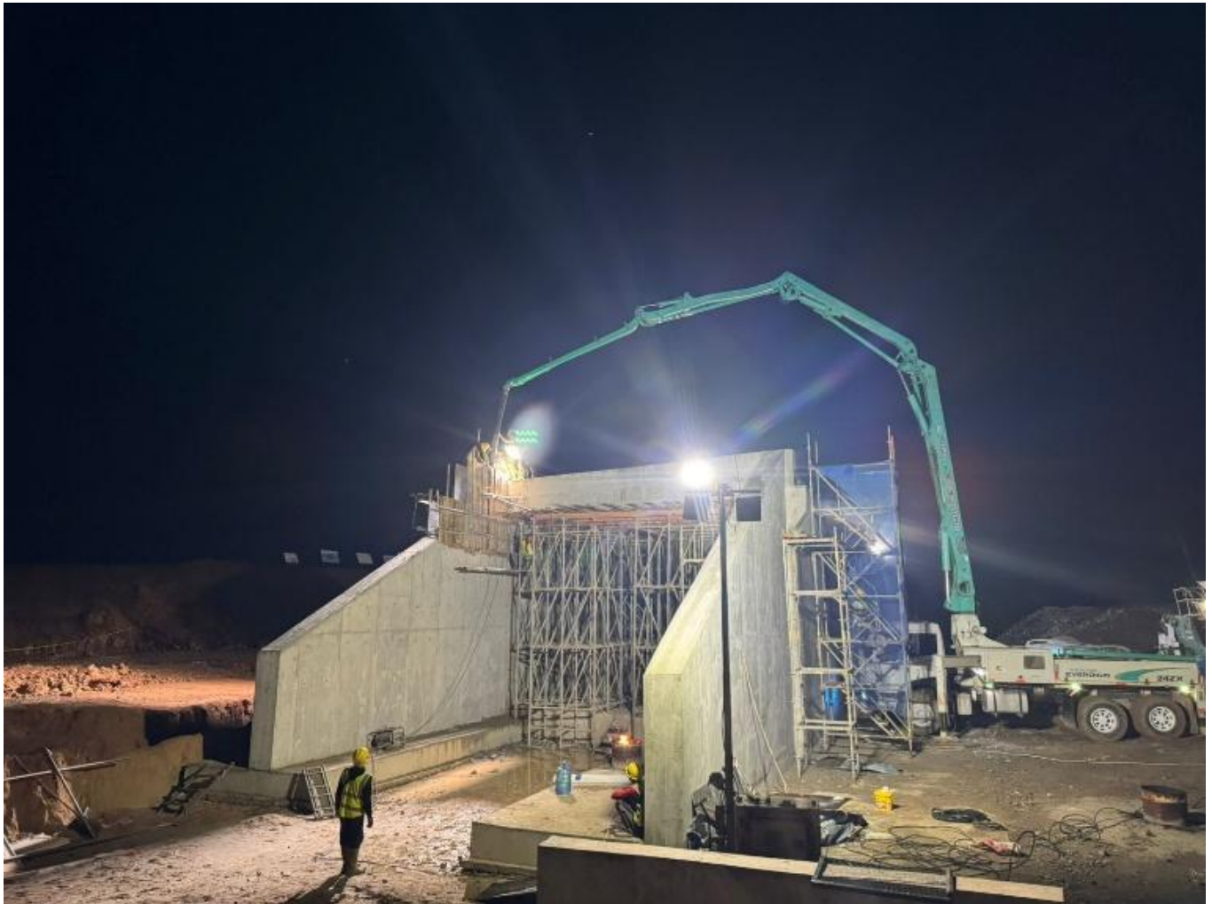
Lampiran 2 Pengecoran Wing Wall Box Culvert STA 68+425
