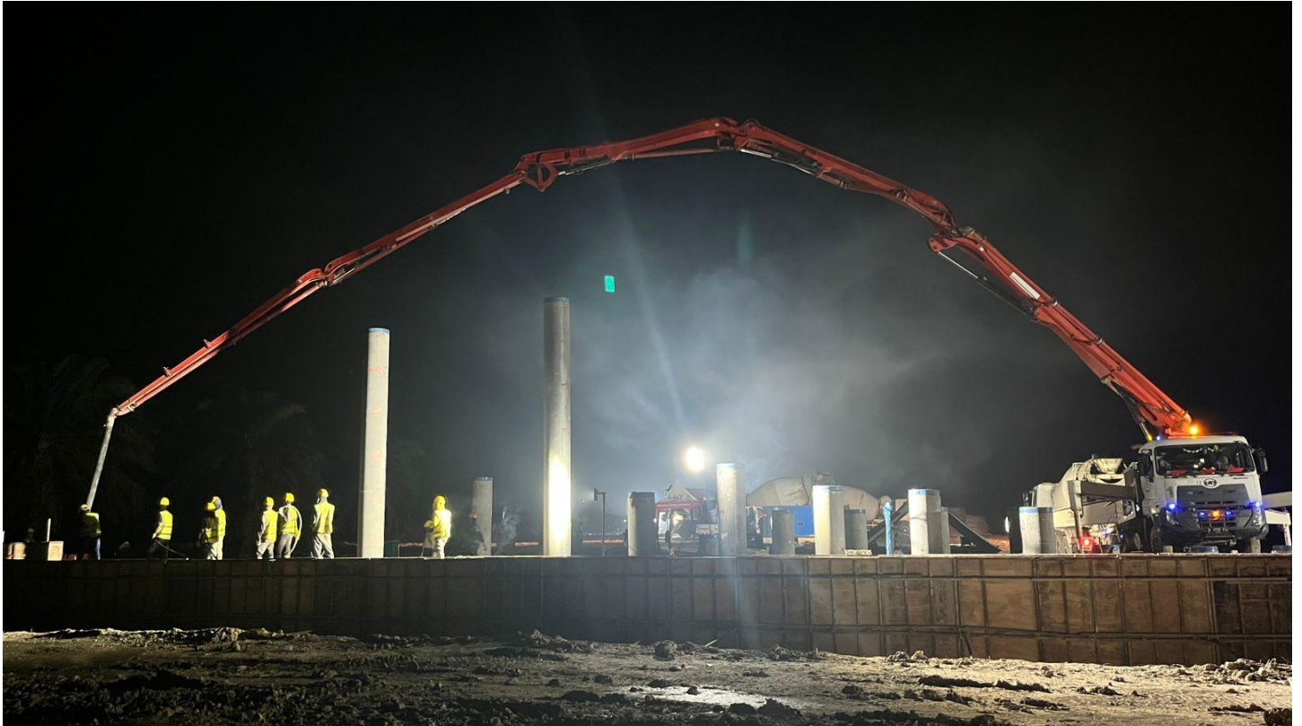
Lampiran 4 Pengecoran Top Slab & Wing Wall Box Culvert STA 81+175
