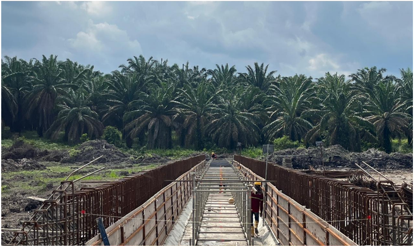
Lampiran 3 Pemasangan Perancah Box Culvert STA 81+086
