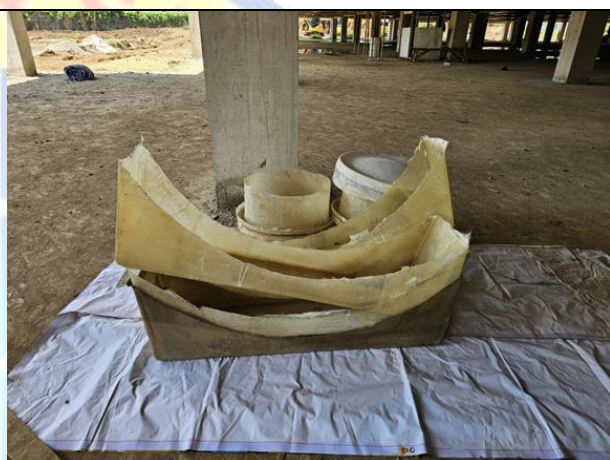
Material Dudukan IPAL Biofilter
