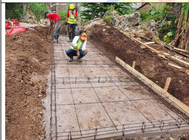
Pembesian Pondasi IPAL Biofilter
