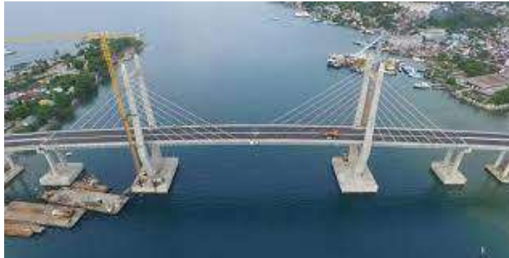
Gambar 2.7 Jembatan kabel ( cable stayed bridge )
