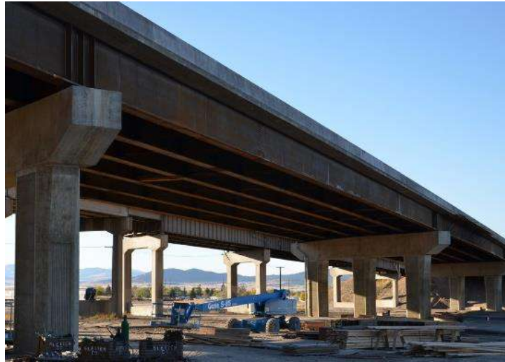
Gambar 2.3 Jembatan gelagar ( girder bridge )
