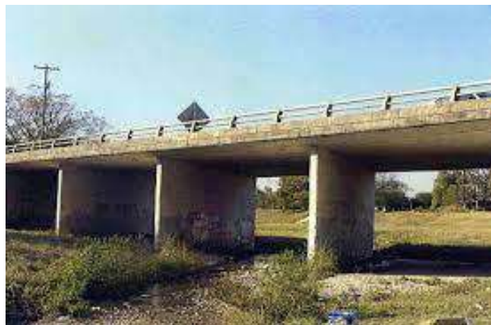
Gambar 2.1 Jembatan Pelat ( slab bridge )
