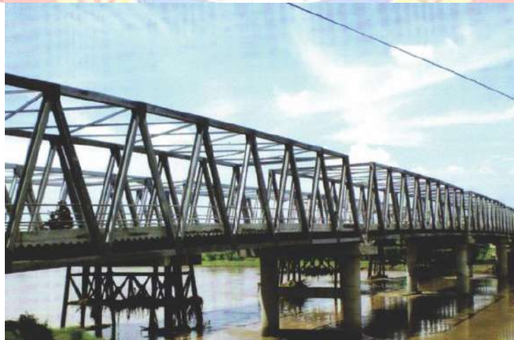
Gambar 2.4 Jembatan rangka ( truss bridge )
