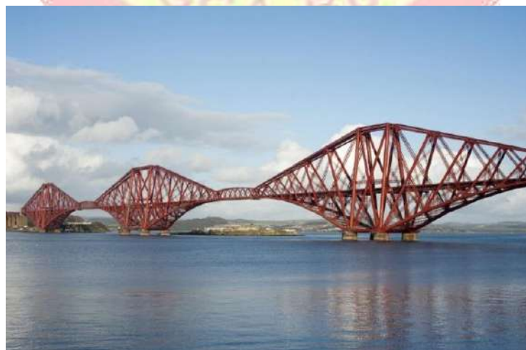
Gambar 2.8 Jembatan cantilever ( cantilever bridge )
