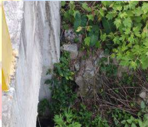
Dinding Penahanan Tanah A2 (Abutmen)
