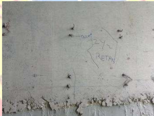
Dinding Tegak A2 (Abutmen)
