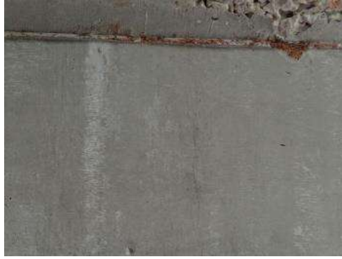
Dinding Tegak A1 (Abutmen)
