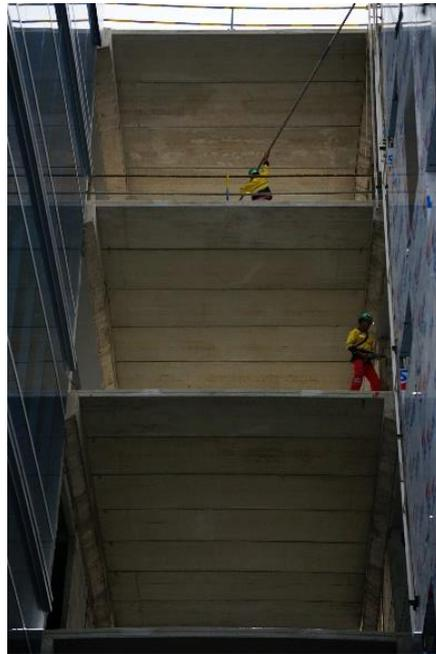
**Gambar 1.1** Pemasangan *Hollow Core Slab*
