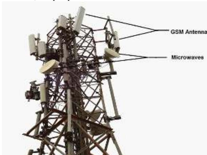
*Gambar 1. 1 Antena Microwave & GSM*
