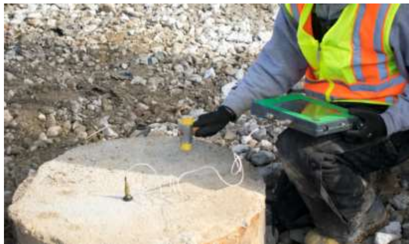
Gambar 2. 16 Pile Integrity Test
