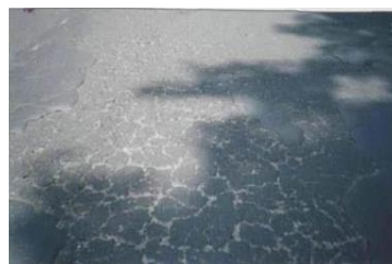
Gambar 2. 22 Pengelupasan ( Weathering and Ravelling )
