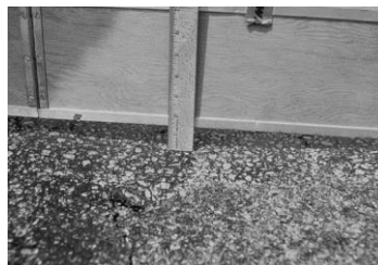
Gambar 2. 18 Alur ( Rutting )
