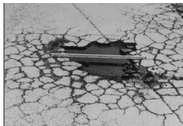
Gambar 2. 16 Lubang ( Potholes )
