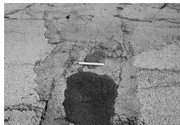
Gambar 2. 14 Tambalan ( Patching and Utility Cut Patching )
