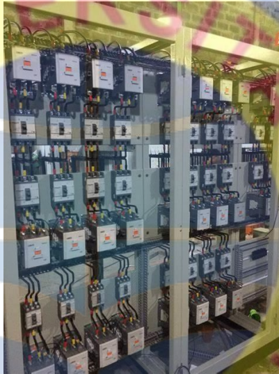
Gambar 2.5 Panel Kapasitor Bank
