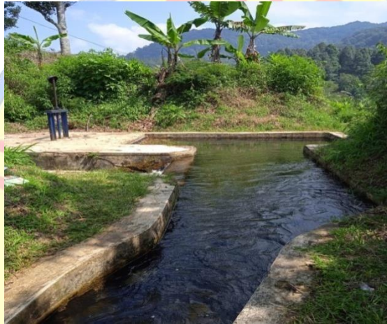
Gambar 2.4. Head Tank (Bak Penenang)
