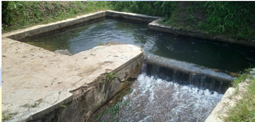
Gambar 2.2. Settling Basin (Bak Pengendap)
