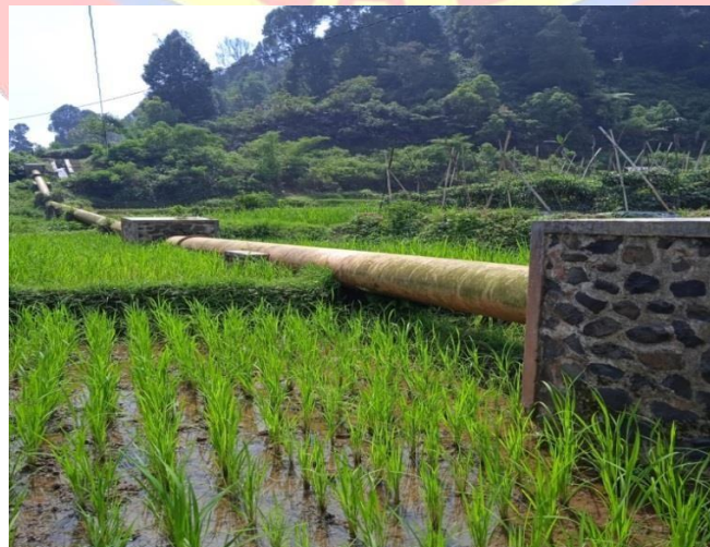
Gambar 2.5. Penstock (Pipa Pesat/ Penstock )
