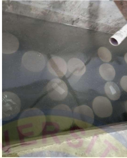
Gambar 4.7 Proses Curing Beton
