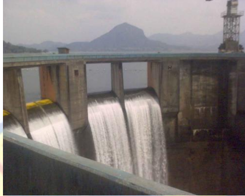
Gambar 3. 14 Pelimpas ( Spillway ) (Doc. Pribadi).
