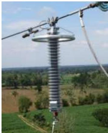
**Gambar 2. 34** Transmision Line Arrester (TLA) (PT. PLN, 2014)
