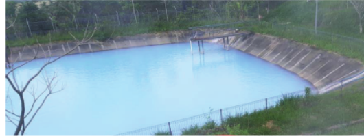
Fig. 5. Ulubelu Geothermal Cooling Pond
