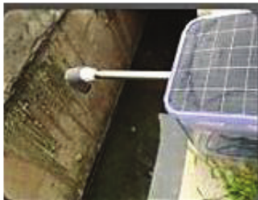
Fig. 11. Placement of transmitter module
